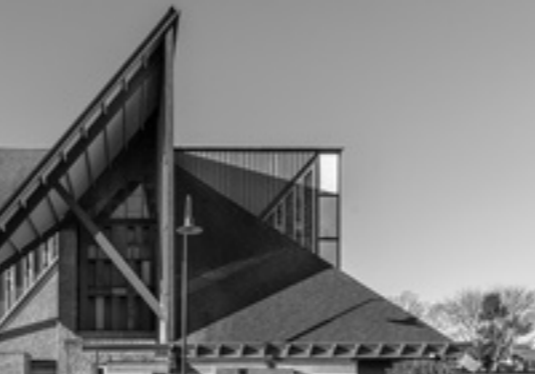
Aotearoa New Zealand: Futuna Chapel, saved from demolition by the trust that purchased it in 2003. Image: Paul McCredie
