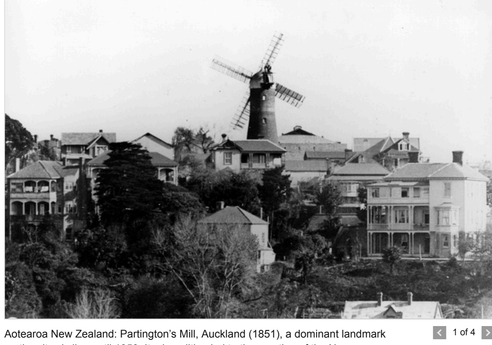
Aotearoa New Zealand: Partington's Mill, Auckland (1851), a dominant landmark on the city skyline until 1950. Its demolition led to the creation of the New Zealand Historic Places Trust. Image: Henry Winkelmann
